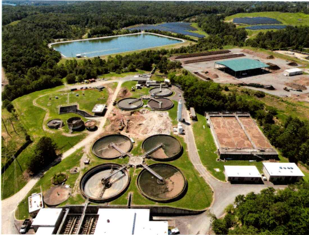
Overview - Construction Area for New Clarifier – Davidson Drive Wastewater Treatment Plant
