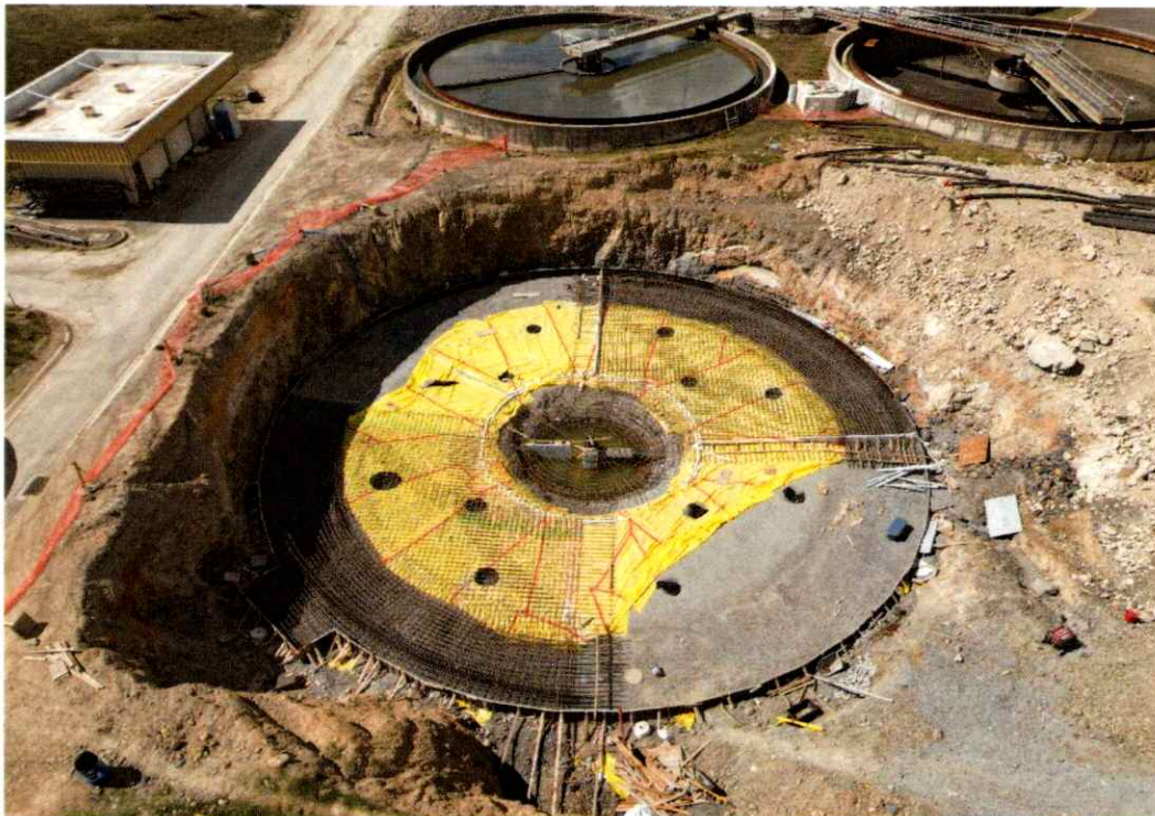
New Clarifier Construction Underway – Davidson Drive Wastewater Treatment Plant
